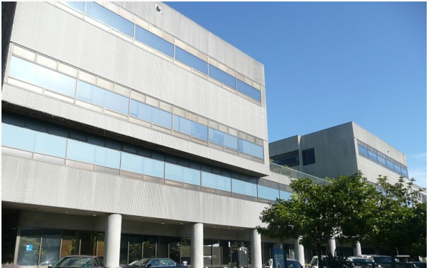
Alta Bates at 2450 Ashby Ave.: the hospital needs to meet seismic standards by 2030 and is considering its options on whether to close, or retrofit/rebuild.. Photo: Frances Dinkelspiel
